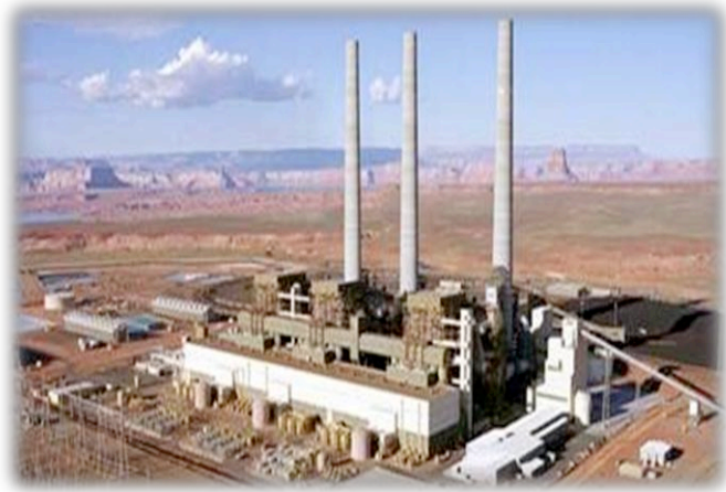
Navajo Generating Station, Page, AZ
