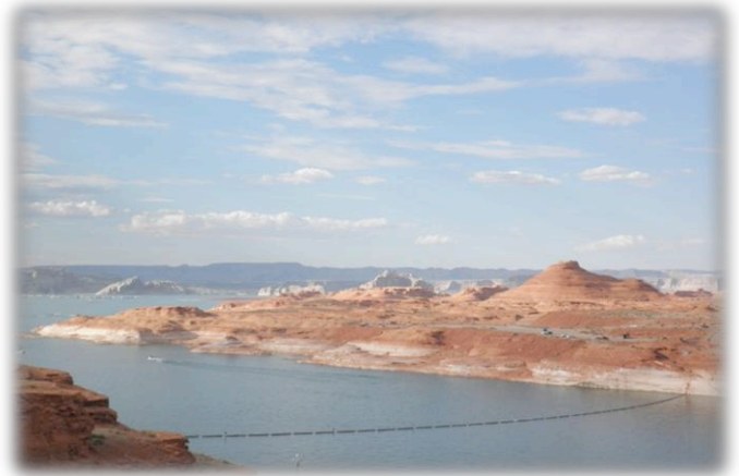
Glen Canyon Dam, Colorado River
