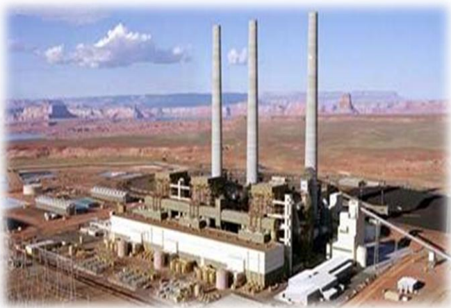
Navajo Generating Station, Page, AZ
